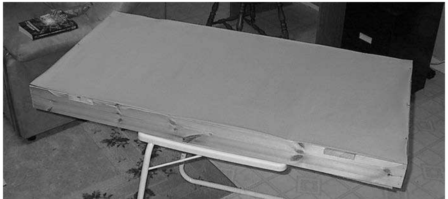
Figure 9.4 Fiberglass panel backing installed.
