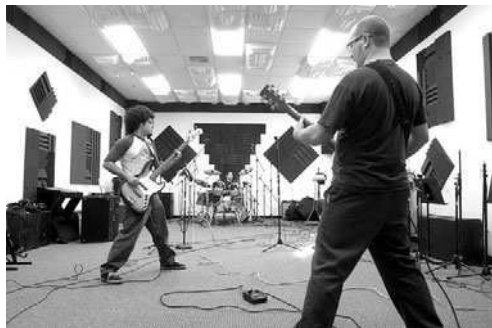
Figure 9.37 Acoustically treated live recording room (courtesy of the Fender Museum).
