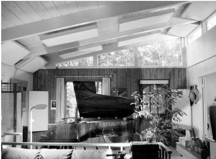
Figure 9.42c MiniTraps installed in living room.
